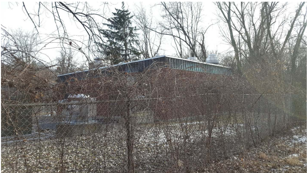
Photo 2. View southeast of a Rensselaer County Sewer District building from the 1970s located within the Study Area.
