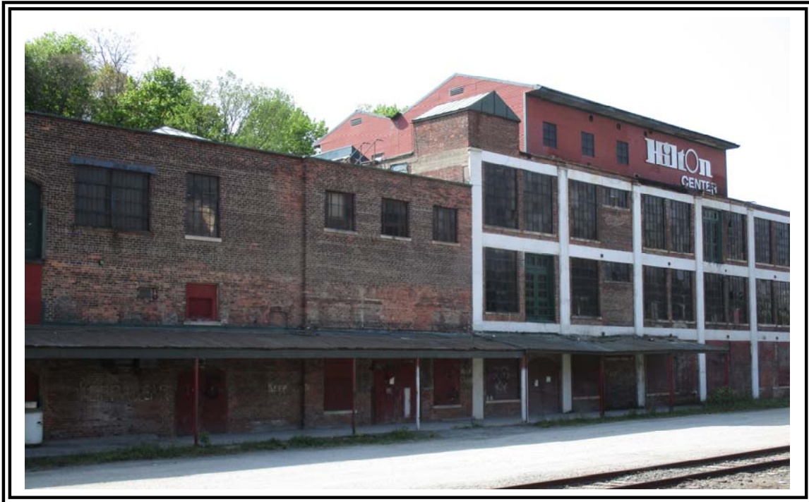
Photo 5-Hilton Center from Boat Launch parking area
