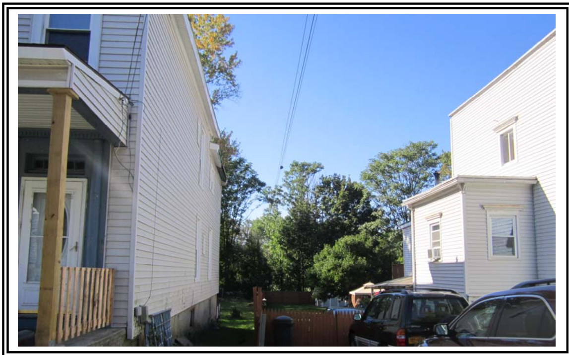
Photo 12-View from Broadway at intersection with MacNaughton Avenue
