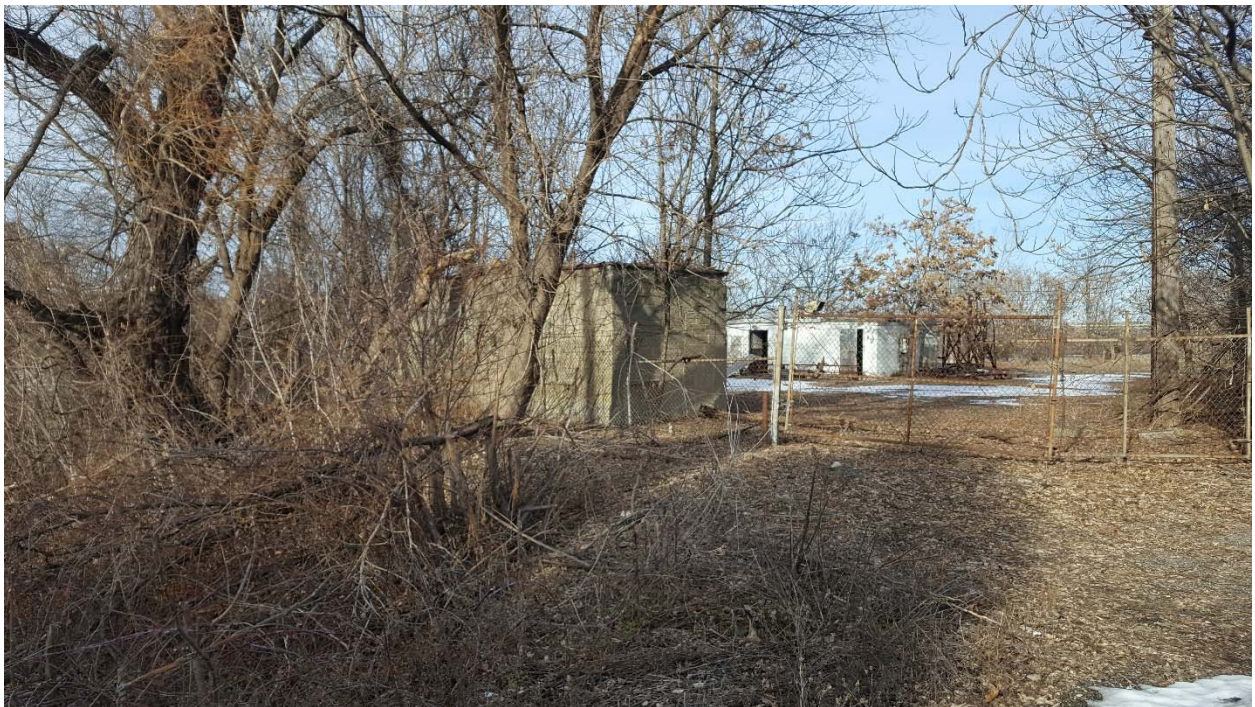
Photo 8. View north of the site of the former Larner Terminal Corporation, which included two large oil storage tanks with capacities of 500,000 and 1 million gallons.
