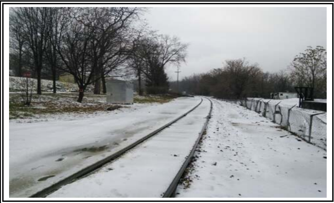
Photo 12 – View looking north along the railroad tracks and property boundary.
