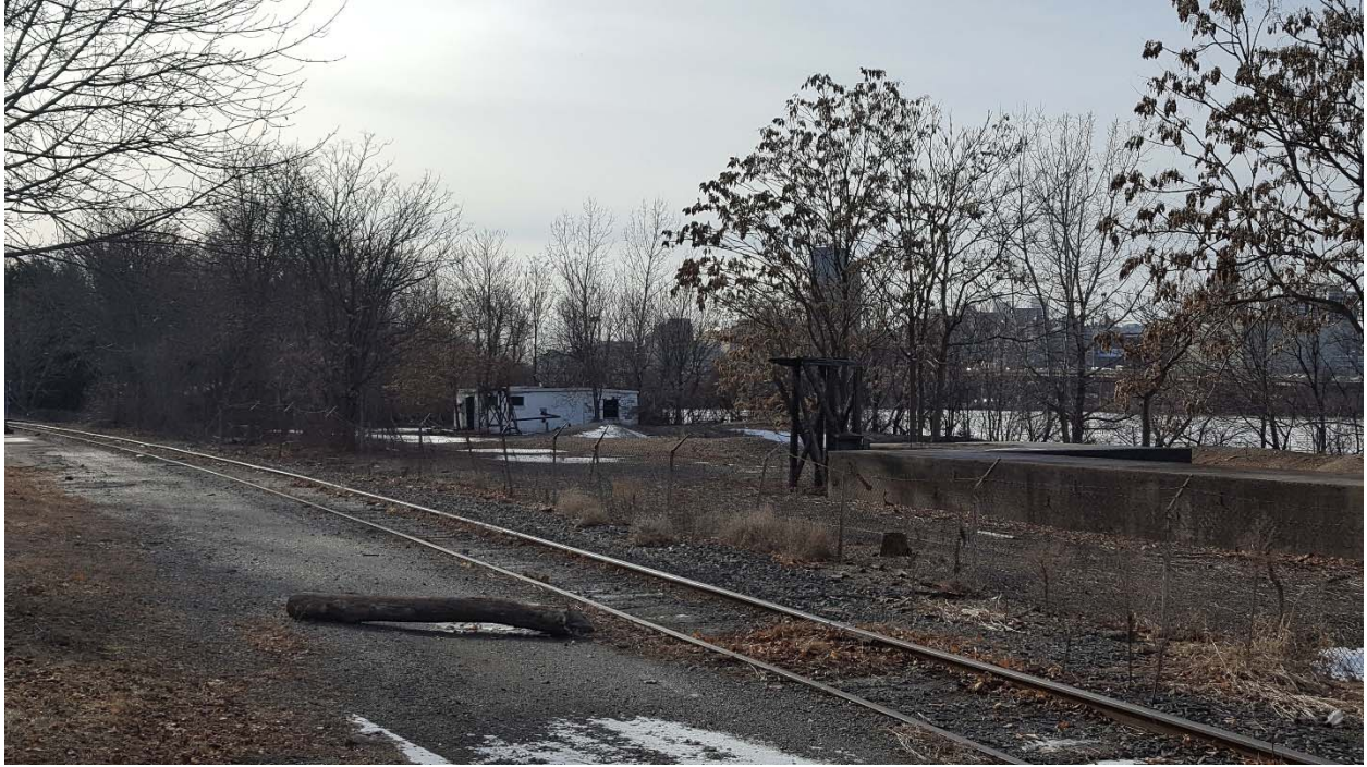
Photo 9. View southwest of the former Larner Terminal Corporation facility.
