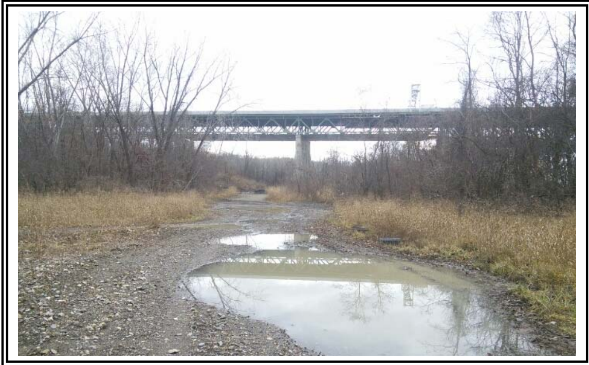
Photo 7-Looking towards Patroon Island Bridge from site interior
