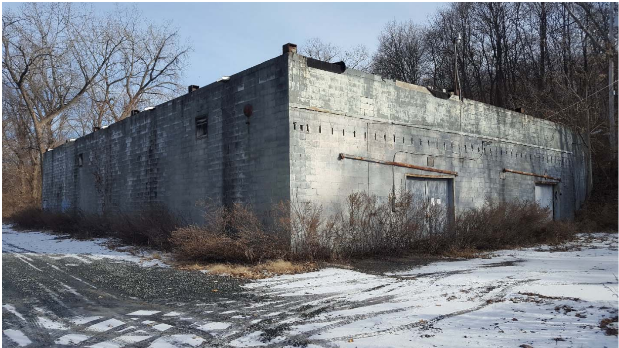
Photo 18. View east of a circa 1950 concrete block garage.
