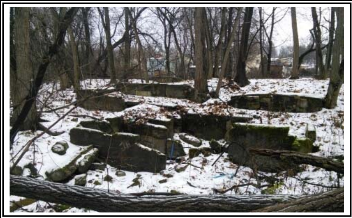
Photo 5 – Remains of a building.
